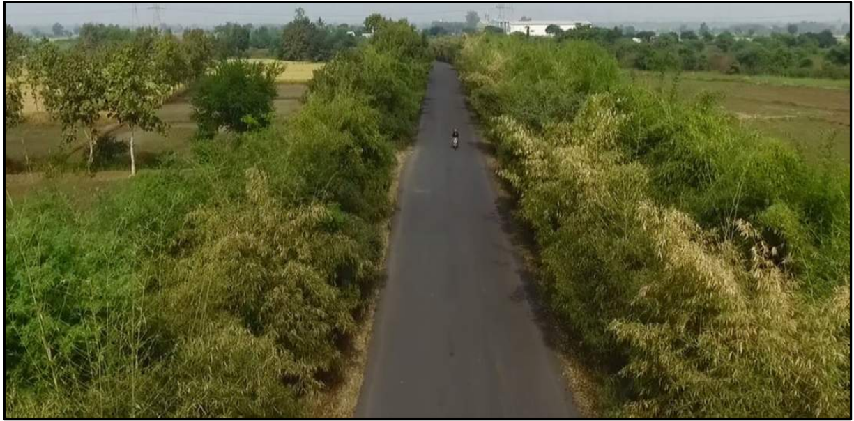
Coal transportation Road, Gondagaon OC, Nagpur Area
