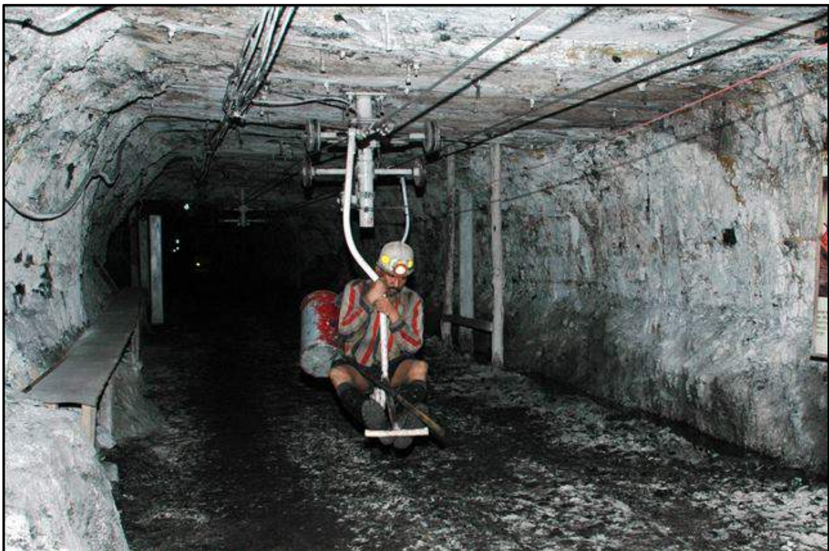
Man-riding system at WCL UG mine
