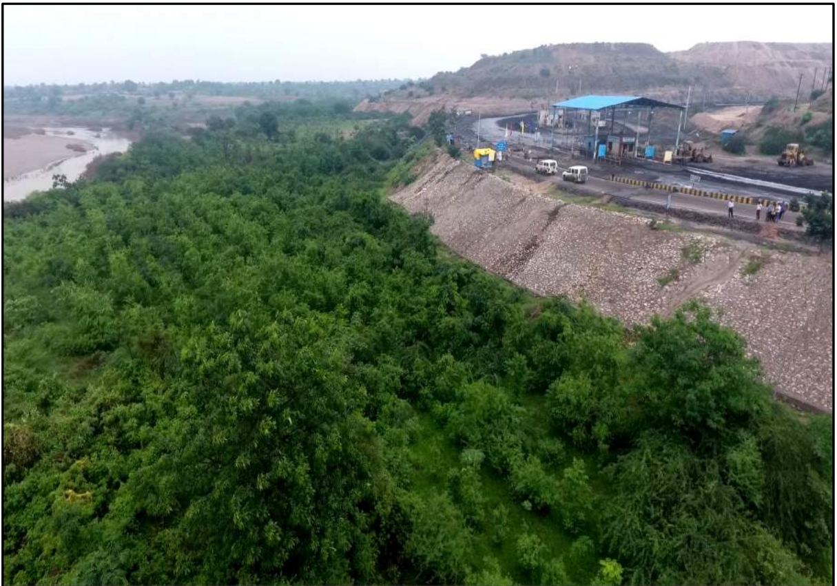
Plantation and stone pitching of embankment at Penganga OC
