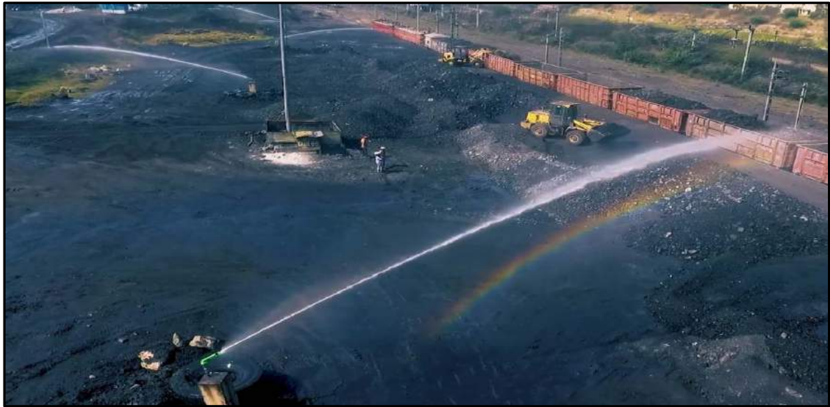
Fixed sprinklers at Coal stock yar, Umrer OC
