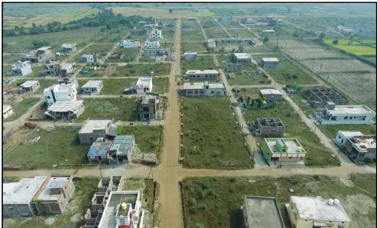
Rehabilitation and resettlement efforts at Gondgaon OCM
