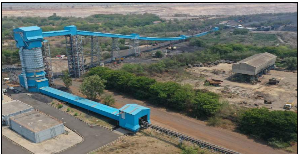
Pipe Conveyor from Bhatadi OC to Chadrapur TPS
