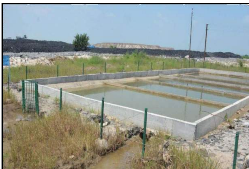
Sedimentation tank, Makardhokra-III UG
