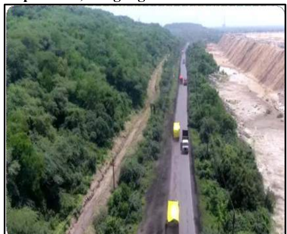
Concrete road, Mungoli
