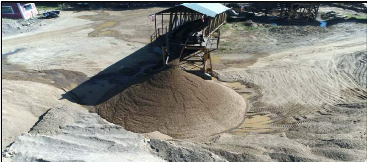
Sand segregation pilot plant at Bhanegaon OCM
