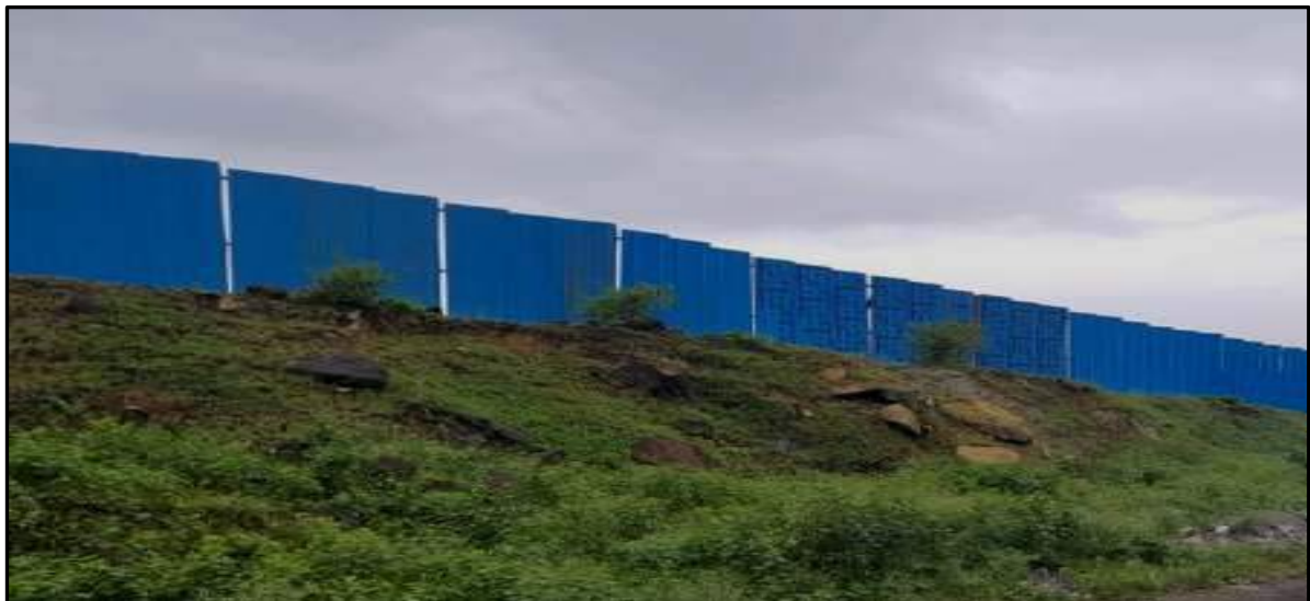
Wind barrier EDC Siding, Pench Area
