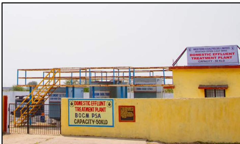
Domestic Treatment plant, Bhatadi OC, Chandrapur Area
